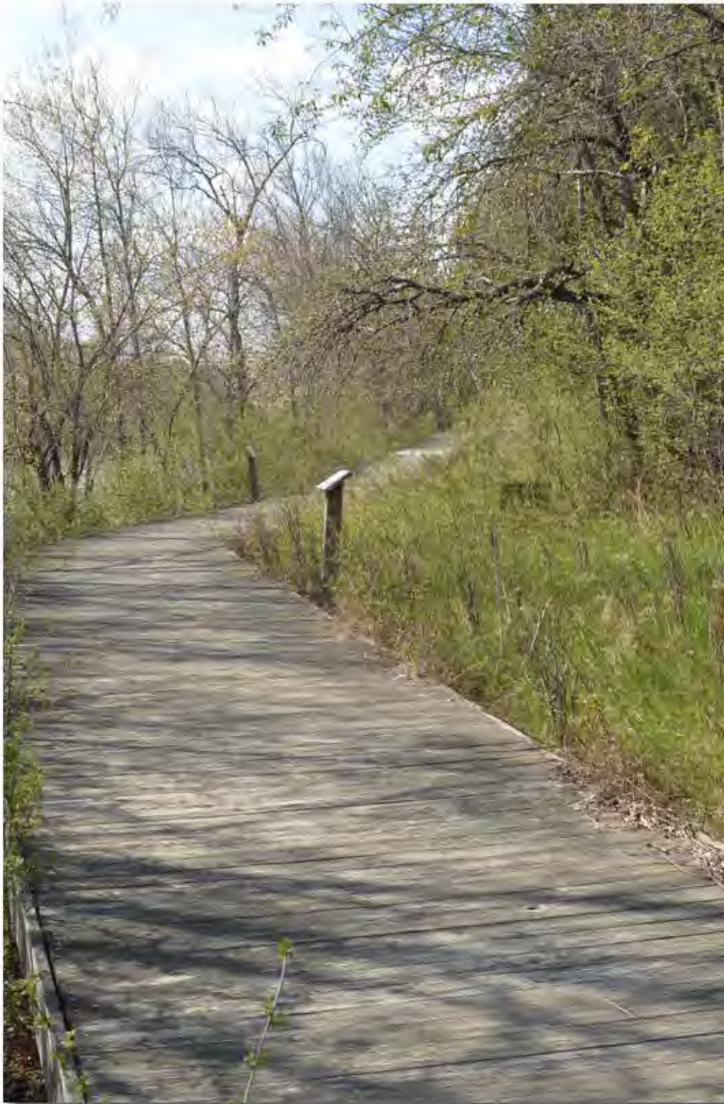
FIGURE 4.7 - BOARDWALK AT LINCOLN PARK
