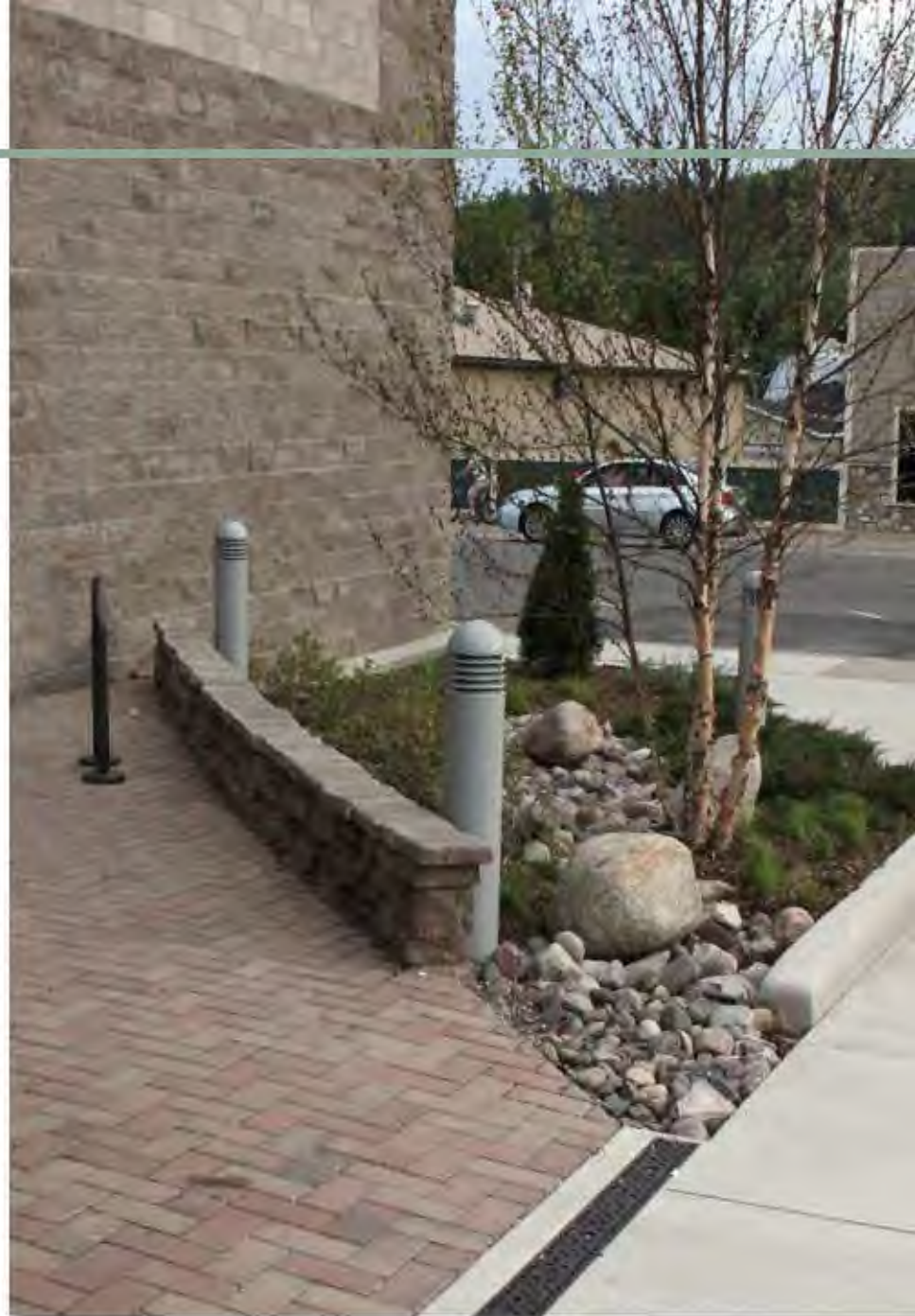
FIGURE 9.3 - BUS STOP IN MUNISING CONVERTED TO UTILIZE POROUS PAVEMENT WITH A RAIN GARDEN
