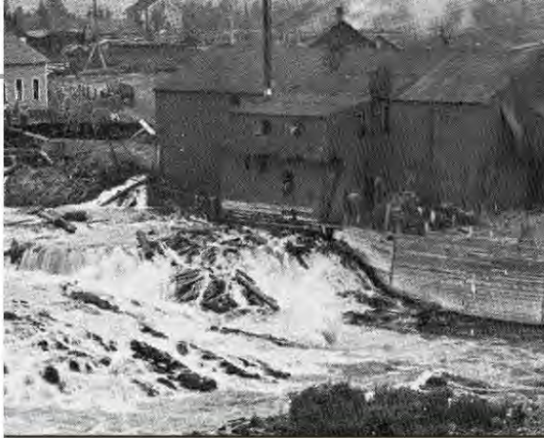
FIGURE 1.1 - PAINT RIVER SAWMILL
