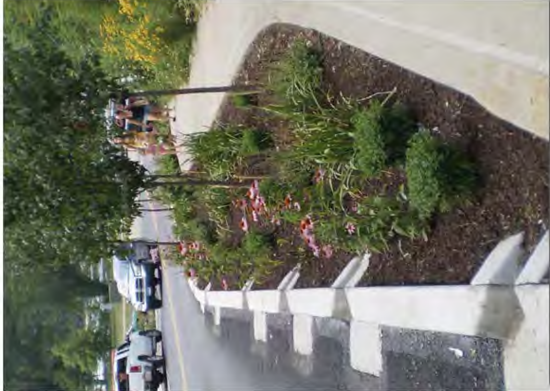
FIGURE 9.2 - STRUCTURAL BMP - DEPRESSED PLANTER COLLECTING STORMWATER FROM THE STREET
