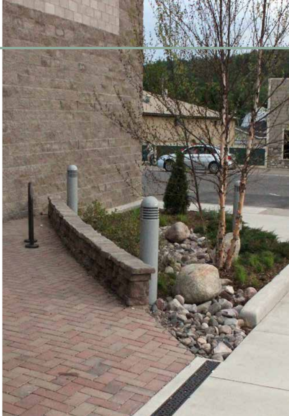
FIGURE 9.3 - BUS STOP IN MUNISING CONVERTED TO UTILIZE POROUS PAVEMENT WITH A RAIN GARDEN
