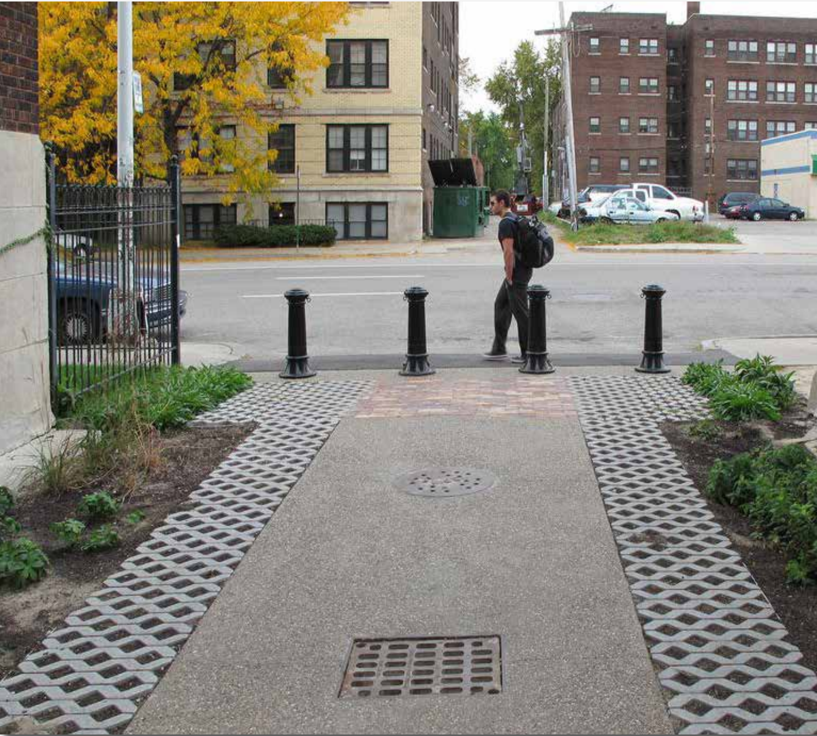
FIGURE 9.5 - EXAMPLE OF A GREEN ALLEY CONVERSION SHOWING BOTH REDUCED PAVEMENT AREAS AND INCLUDING POROUS PAVEMENT
