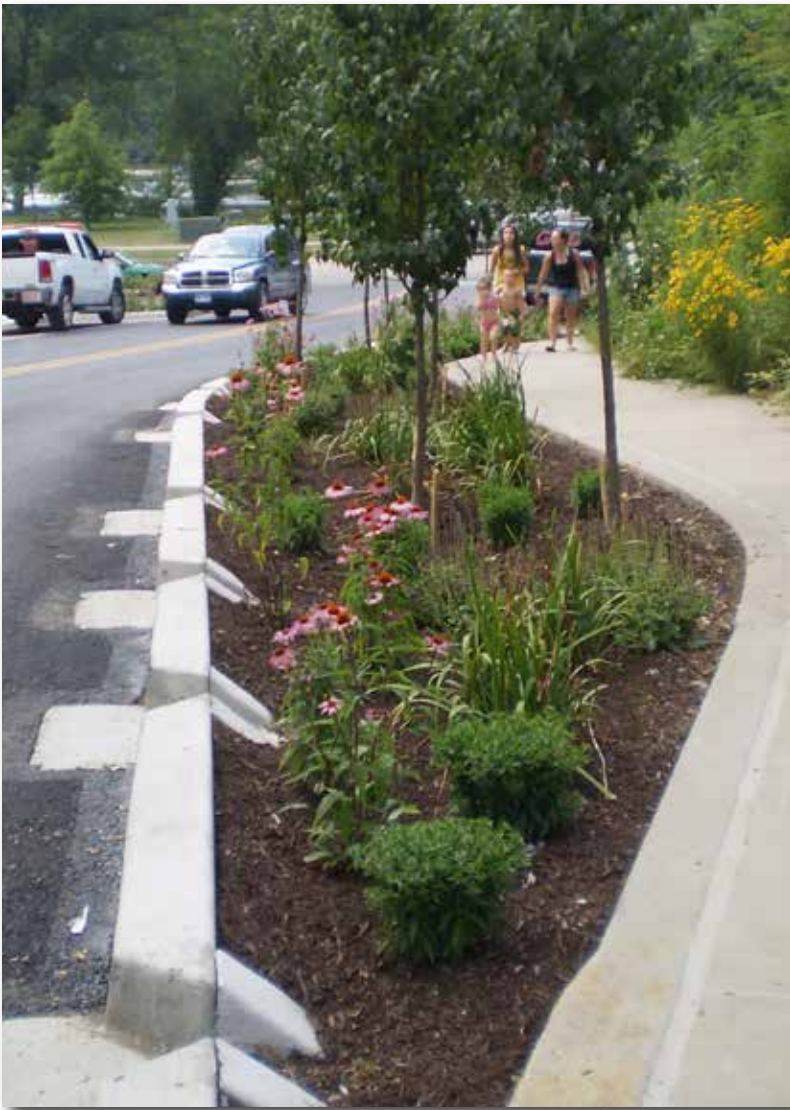
FIGURE 9.2 - STRUCTURAL BMP - DEPRESSED PLANTER COLLECTING STORMWATER FROM THE STREET
